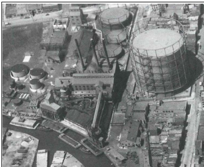
Manufactured Gas Plant at the Gowanus Canal
