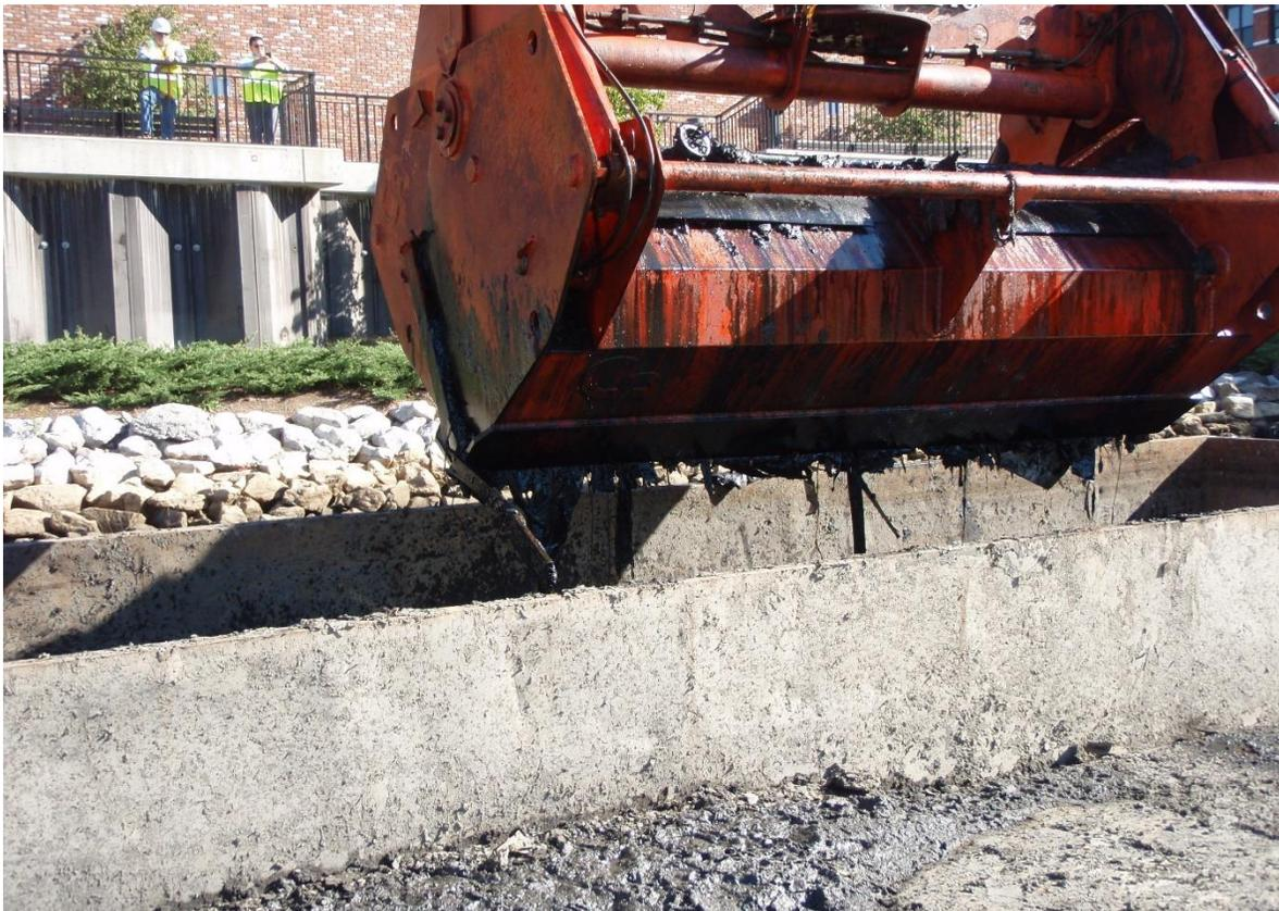
Photograph 2 – TB4 TP4 Dredge Bucket: Note the plastic and modern debris hanging from dredge bucket.
