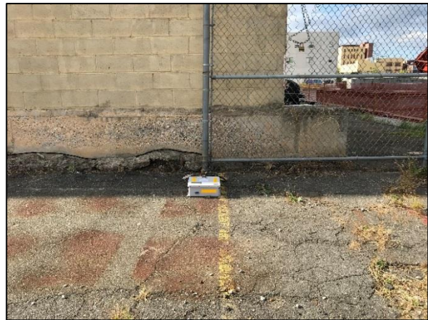
Photo 5: Vibration Monitoring Location VM-2 (12 October 2017)
