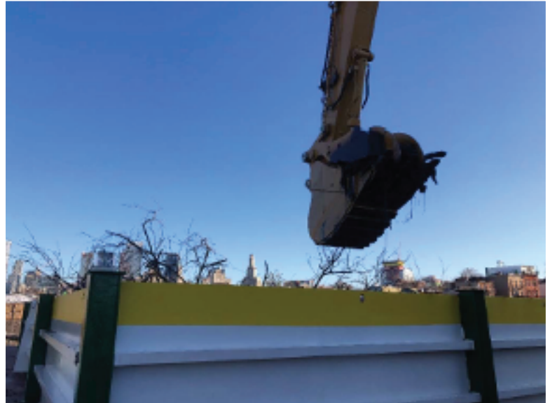
First dredge bucket from RTA1
