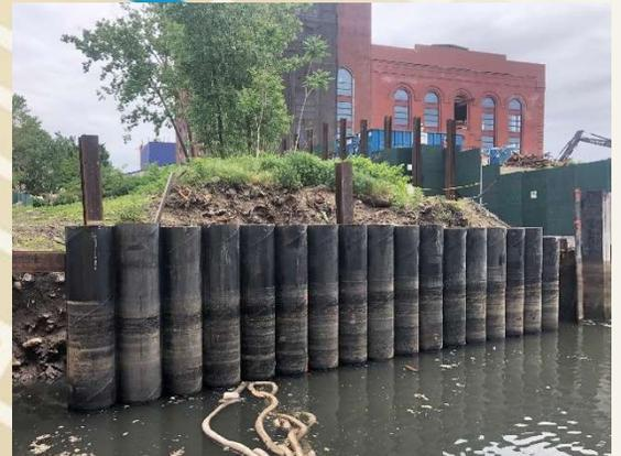
*Pipe pile bulkhead at former 1<sup>st</sup> Street Turning Basin*
