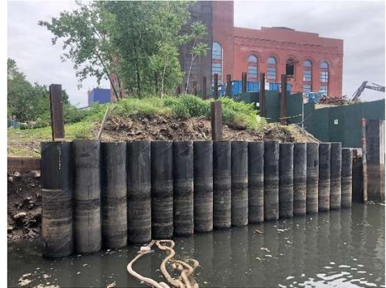
Figure 1: Pipe Pile Bulkhead at the 1<sup>st</sup> Street Turning Basin
