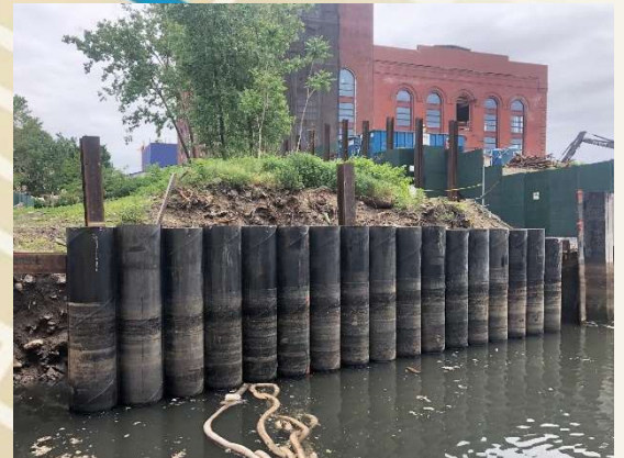
Pipe pile bulkhead at former 1 st Street Turning Basin
