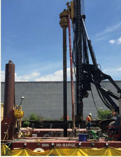
Auger mixing cement into contaminated native sediment during pilot ISS in 7 th Street Turning Basin (conducted in 2015)
