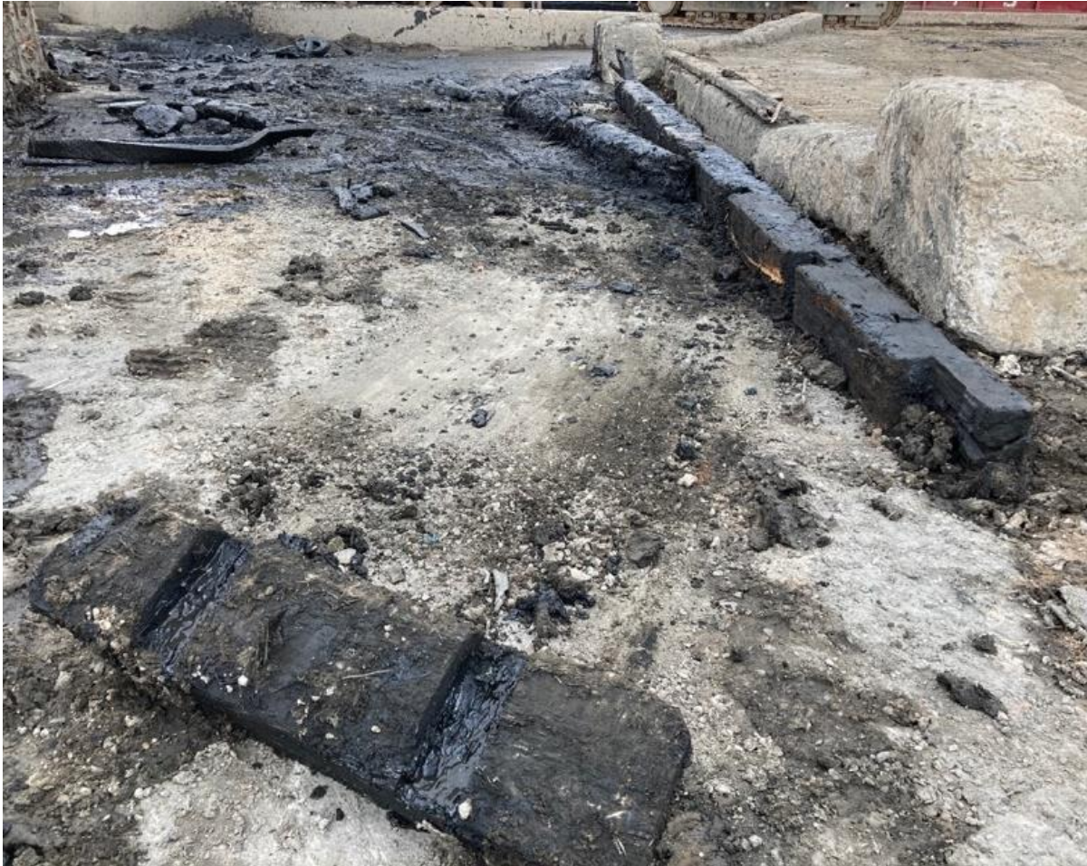
Photograph 4 – Possible bulkhead timbers recommended for discard.
