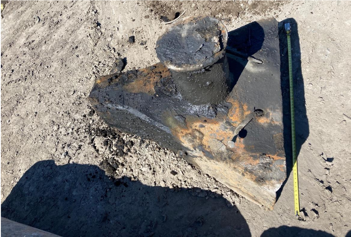
Photograph 3 – View of bollard item, overview.
