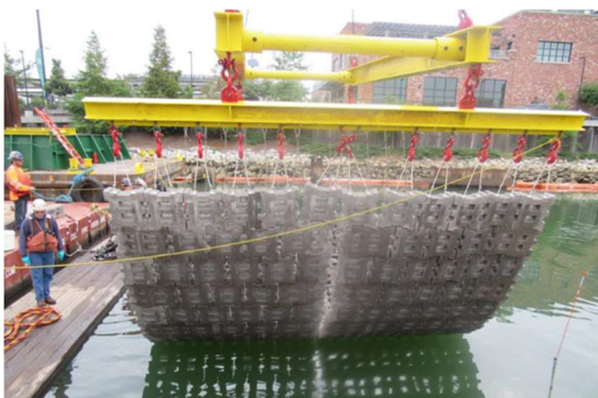
Articulated concrete mat being placed in 4 th Street Turning Basin
