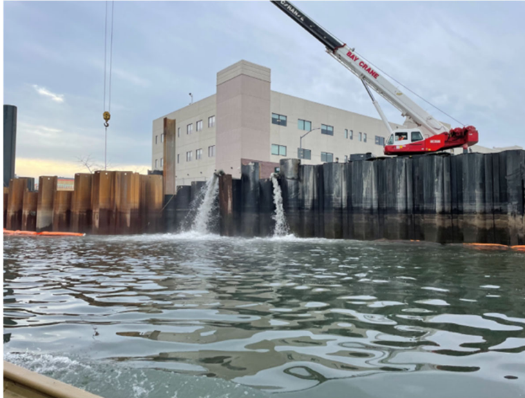
Figure 7. Discharge into the canal unrelated to remedial construction activities was observed from the Salt Lot due to dewatering activities from behind the cofferdam on January 30, 2023.
