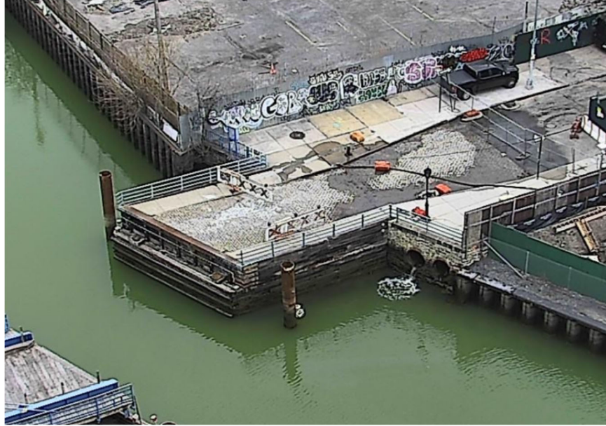
Figure 9. Discharge from high level storm sewer pipe on February 9, 2023 at 3:45 PM.
