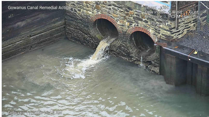
Figure 10. Discharge from high level storm sewer pipe on February 17, 2023 at 10:15 AM during wet weather conditions.
