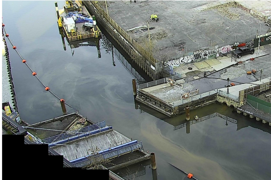
Figure 7. Discharge from high level storm sewer pipe on February 14, 2023 at 4:15 PM during dry weather conditions.
