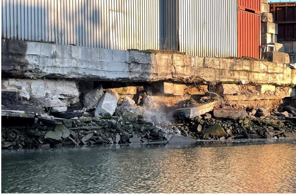
Figure 8. Discharge from concrete plant on March 29, 2023 at 7:30 AM.
