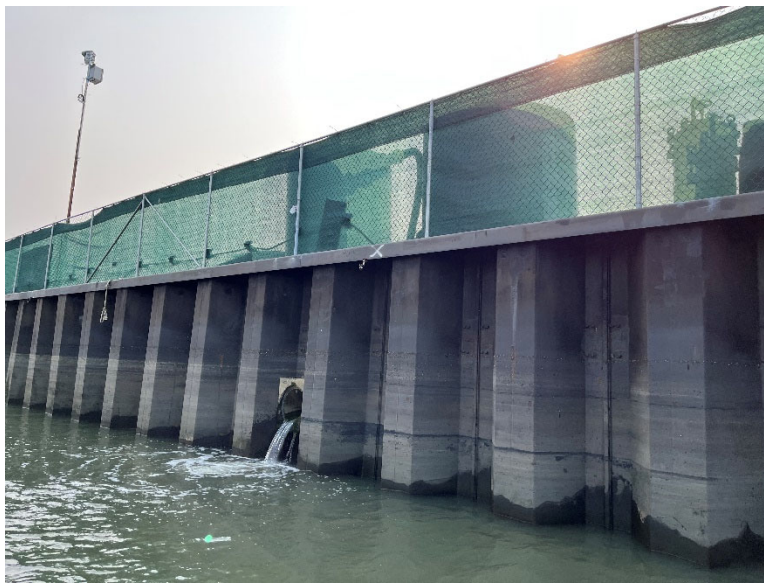
Figure 7. Discharge from the drain at Bayside North on May 22, 2023 at 5:15 PM.
