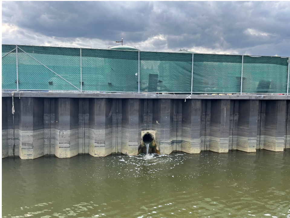
Figure 6. Discharge from the storm water outfall at the Bayside North construction site located between Union Street and Degraw Street on June 5, 2023 at 10:45 AM.
