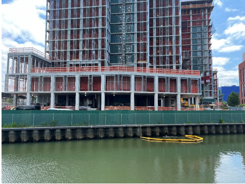
Figure 8. Discharge from the 420 Carrol on June 13, 2023 at 11:15 AM.
