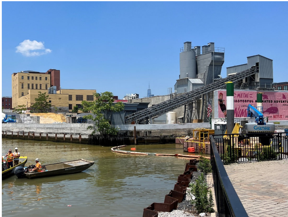
Figure 7. Deployment of turbidity curtain based on visual impacts on July 5, 2023 at 12:00 PM.
