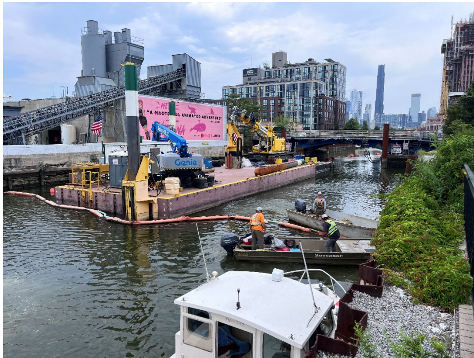
Figure 7. Deployment of turbidity curtain based on visual impacts on July 13, 2023 at 12:30 PM.
