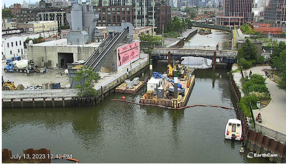
Figure 8. Deployment of turbidity curtain on July 13, 2023 at 12:45 PM.
