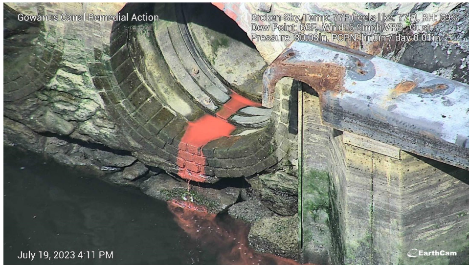
Figure 10. Red discharge from high level storm sewer pipe on July 19, 2023 at 4:15 PM.
