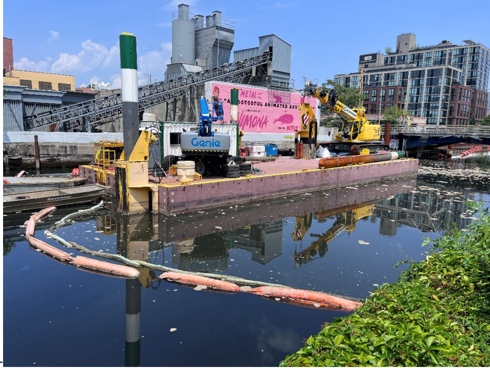
Figure 8. Deployment of turbidity curtain on July 20, 2023 at 12:15 PM.
