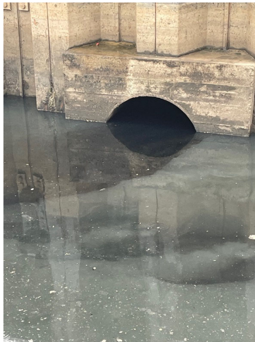
Figure 7. Turbid discharge from high level storm sewer pipe north of Union Street Bridge on August 24, 2023.
