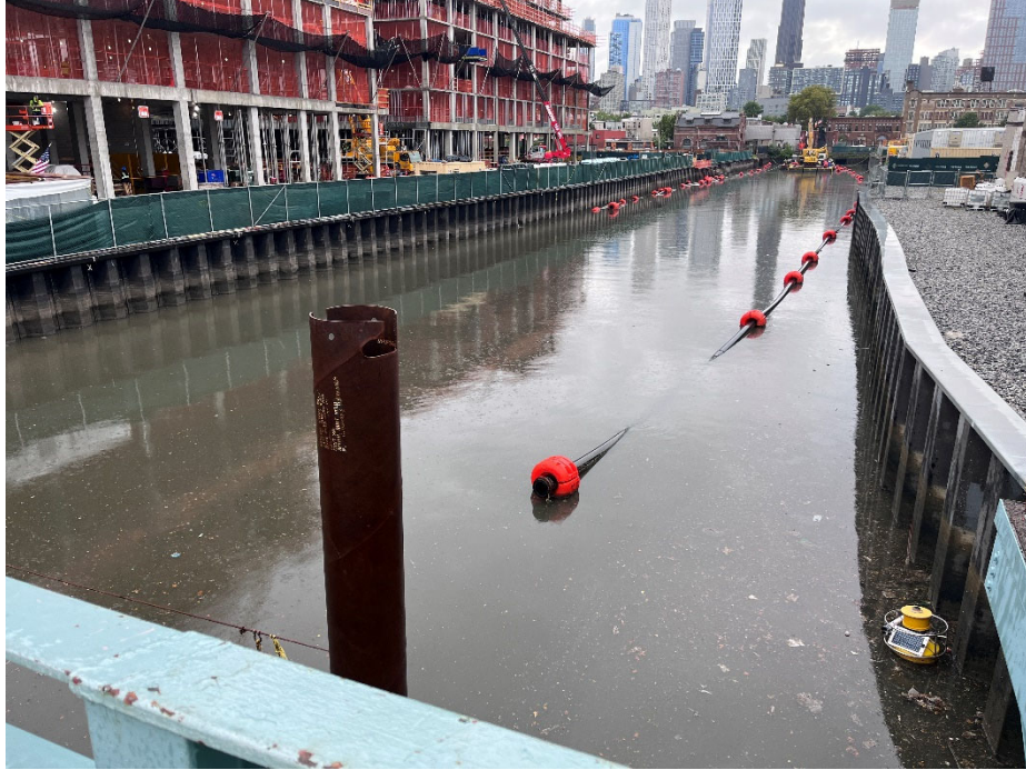
Figure 10. Debris observed north of Union Street Bridge on August 25, 2023 at 9:00 AM.
