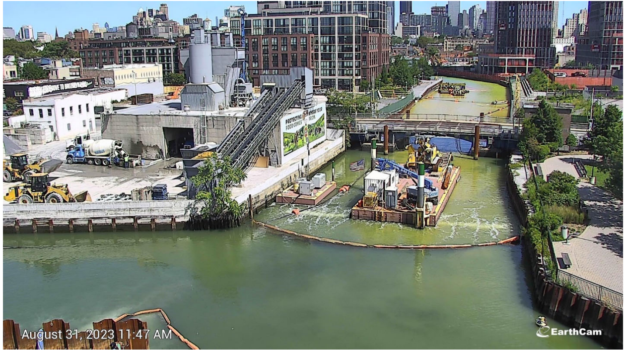
Figure 14. Deployment of the air and turbidity curtain on August 31, 2023 at 11:45 AM.
