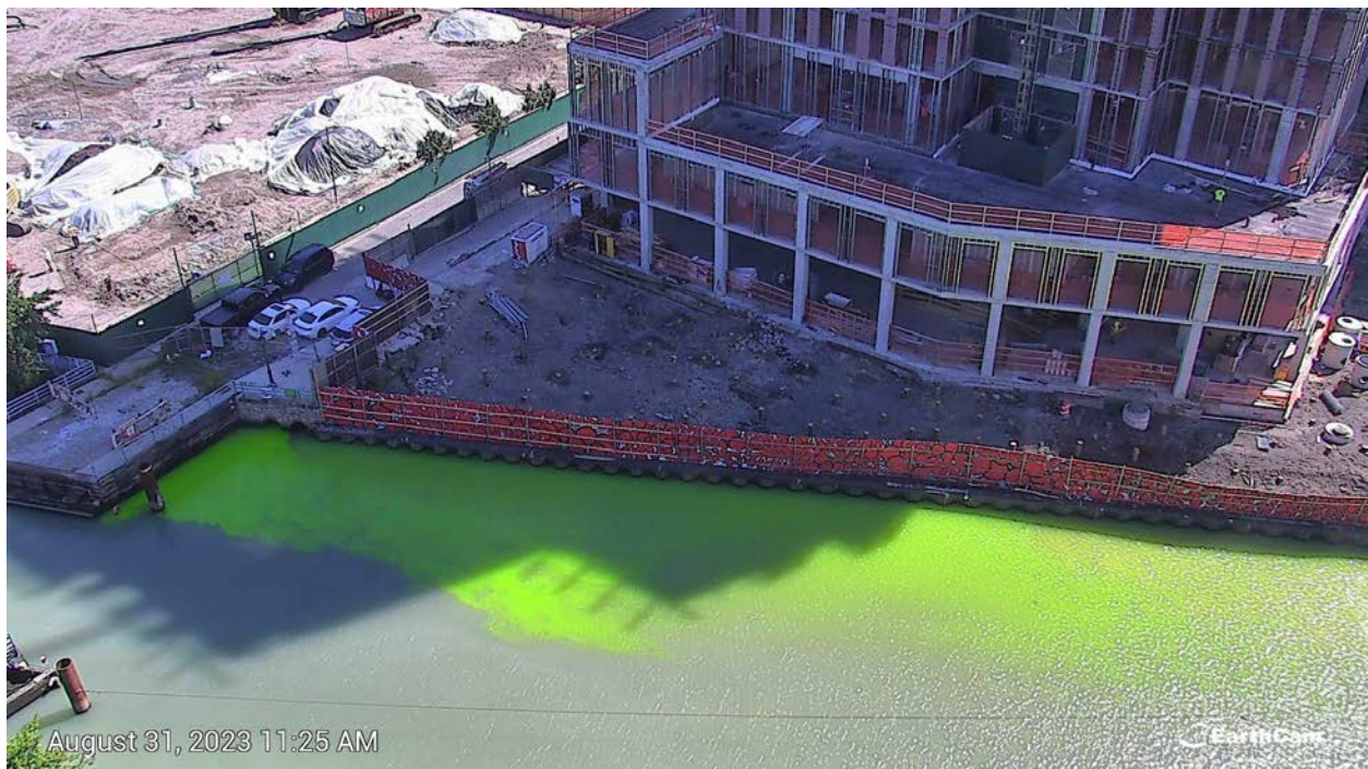
Figure 7. Bright green discharge from high level storm sewer pipe at Carroll Street Bridge on August 31, 2023 at 11:30 AM.
