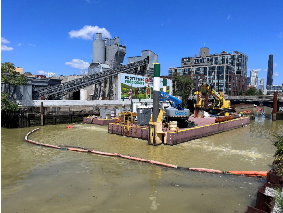
Figure 12. Deployment of the air and turbidity curtain on August 30, 2023 at 12:45 PM.
