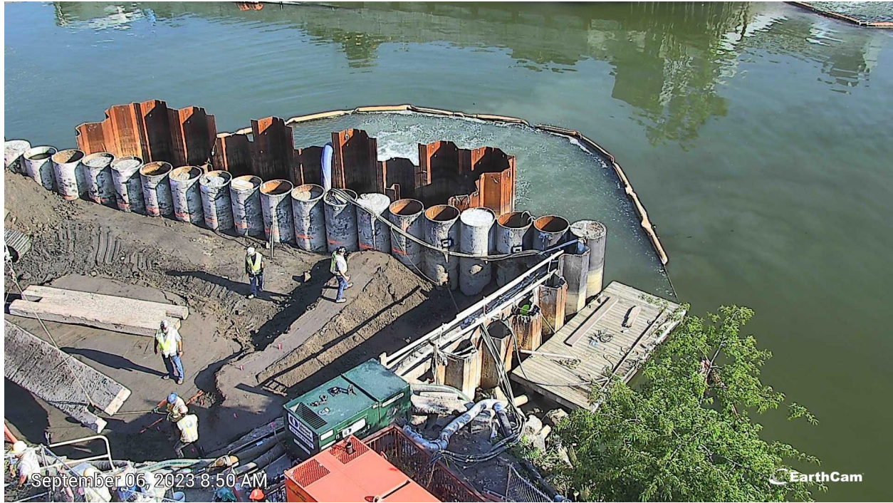
Figure 8. Turbid discharge from the Salt Lot on September 6, 2023 at 8:45 AM.
