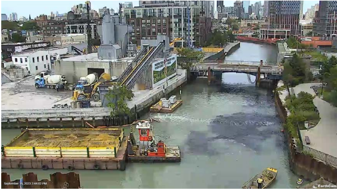
Figure 12. Visual indications of elevated turbidity were periodically observed attributable to resuspension of sediment from prop wash from a passing tugboat pushing a mini-hopper within 100 feet of the sentinel buoys on September 15, 2023 at 2:45 PM.
