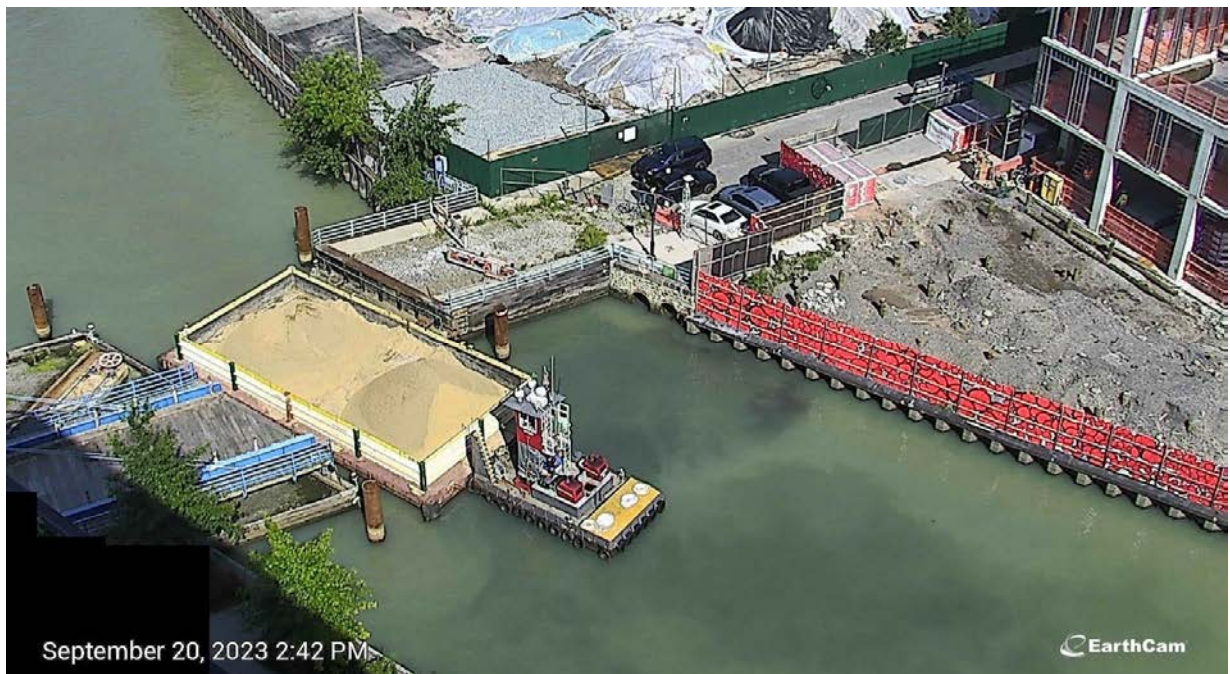
Figure 11. Visual indications of elevated turbidity were observed due to resuspension of sediment from prop wash from a passing tugboat pushing a mini-hopper within 100 feet of the South Carrol St Bridge Sentinel Buoy on September 20, 2023 at 2:45 PM.
