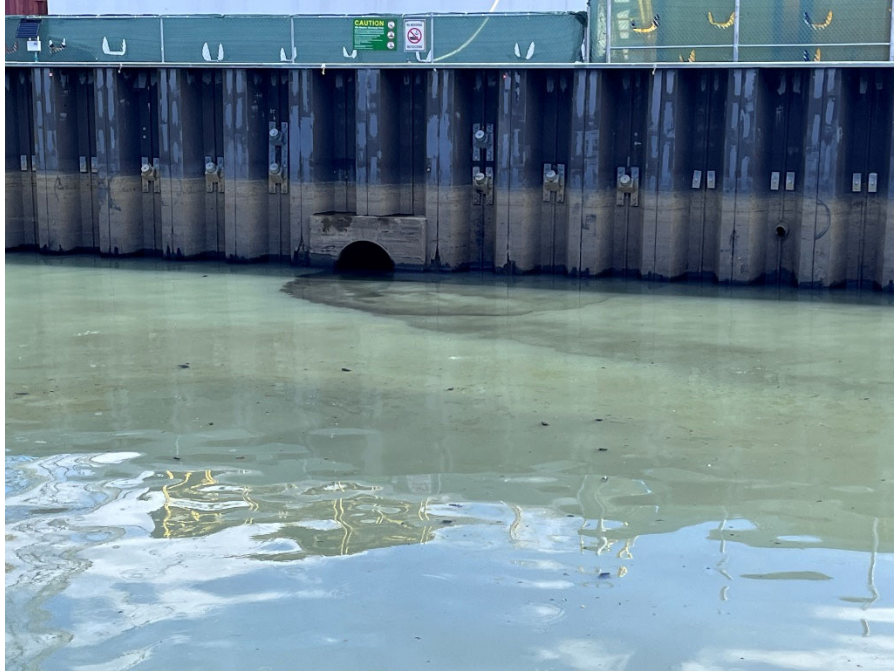
Figure 12. Turbid discharge from the outfall opposite Douglass Street on September 28, 2023 at 10:30 AM.
