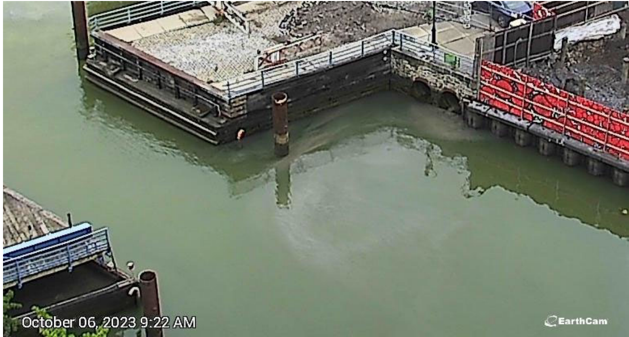
Figure 12. Discharge from high level storm sewer pipe on October 6, 2023 at 9:15 AM.
