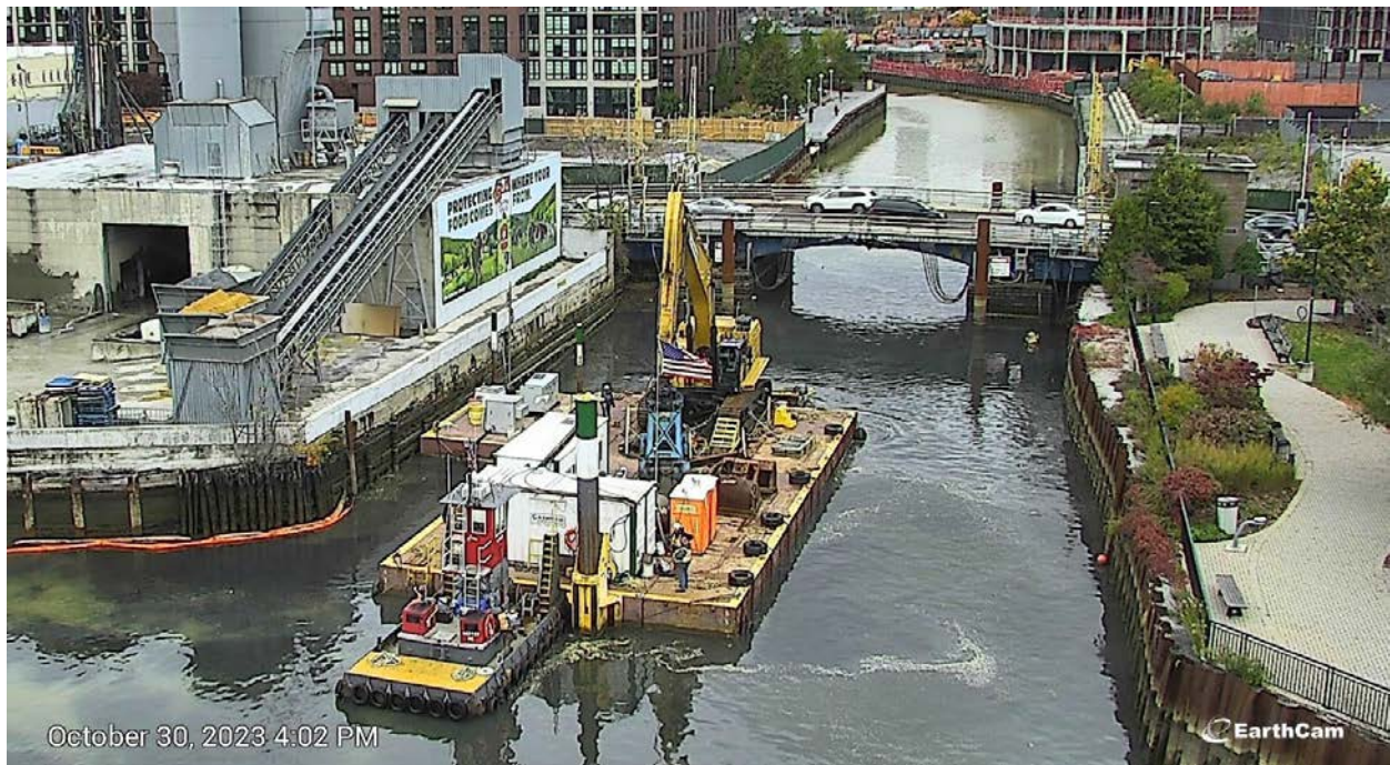
Figure 7. Turbid discharge from temporarily suspended sediments from passing vessels on October 30, 2023 at 4:00 PM.
