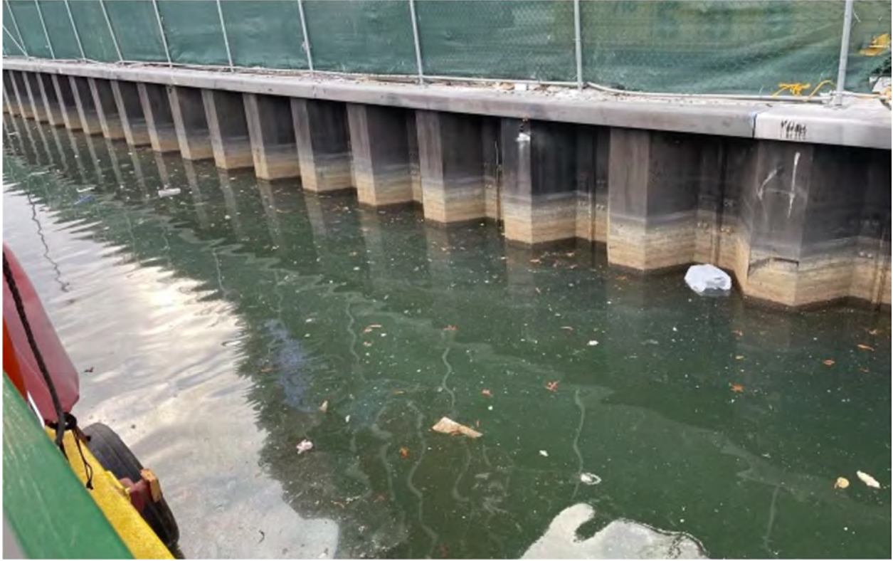
Figure 10. Excessive debris observed in the north pool between the headwall and Union Street Bridge on December 6, 2023.
