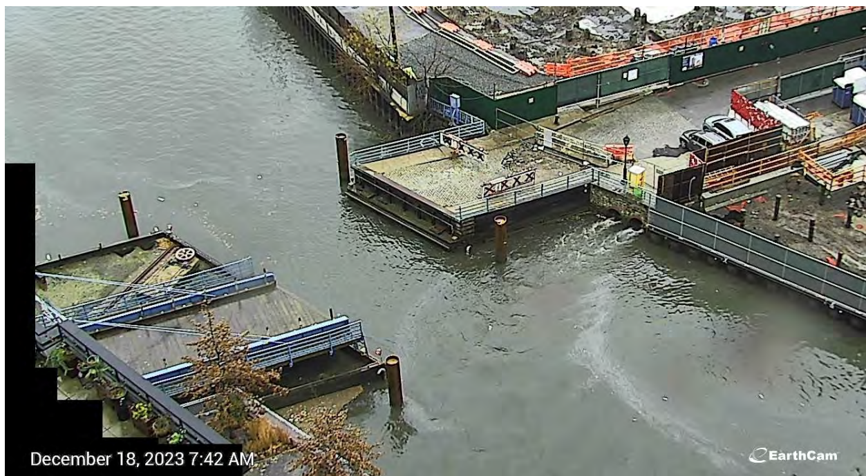
Figure 7. Turbid and sheen discharge from the high-level storm sewer pipe adjacent to OH-005 on December 18, 2023 at 7:45 AM.
