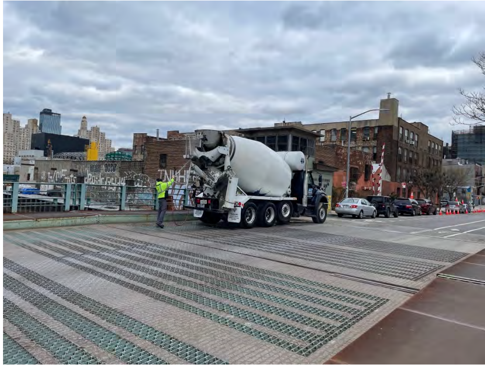
Figure 8. Discharge at the Union Street Bridge from concrete truck related to the northern Presidents Street property on Wednesday, January 10, 2024.
