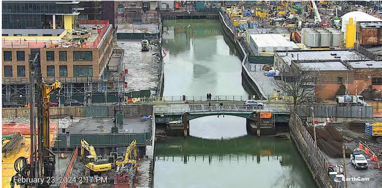
Figure 9. On the afternoon of Friday, February 23, 2024, a sheen was observed around Union Street Bridge migrating south with still wind conditions and an incoming tide.
