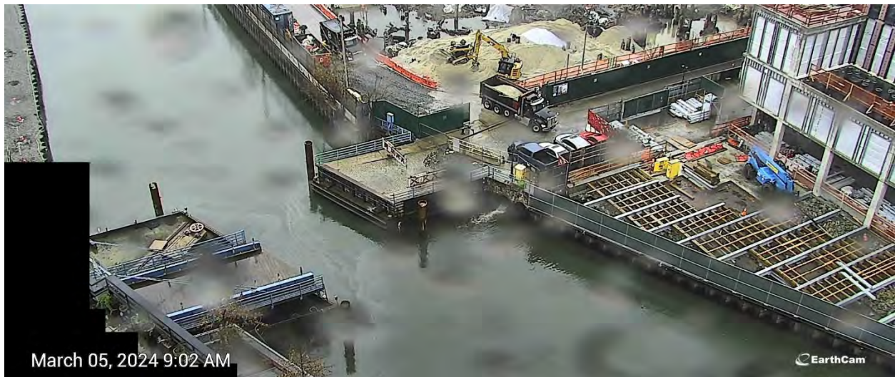
Figure 9. Turbid discharge from high level storm sewer pipe on March 5, 2024 at 9:00 AM.
