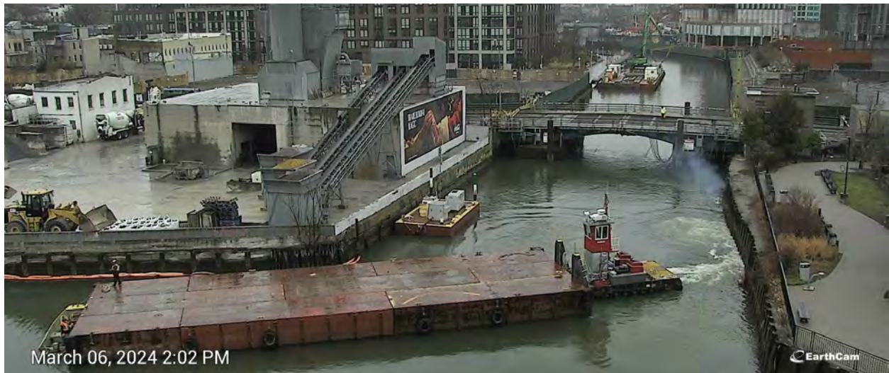
Figure 10. Vessel (used for transporting a barge previously loaded with ACB Mats) moving through Third Street Bridge at approximately 2:00 PM on March 6, 2024.
