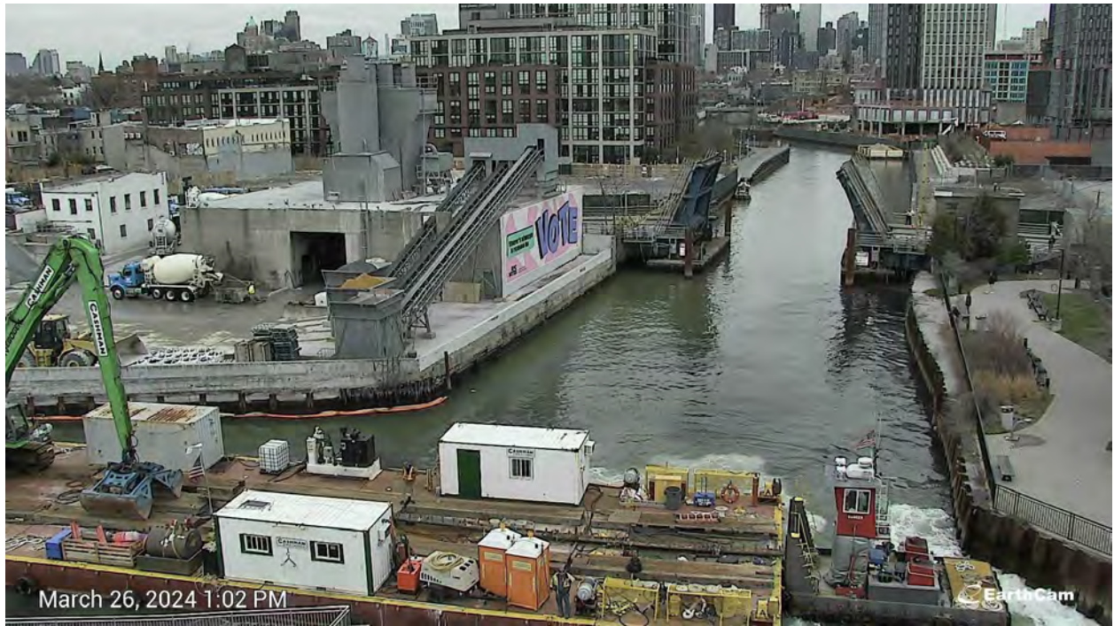
Figure 10. Visual indication of elevated turbidity outside RTA1 as a result of temporarily suspended sediments from passing vessels at 1:00 PM on Tuesday, March 26, 2024.
