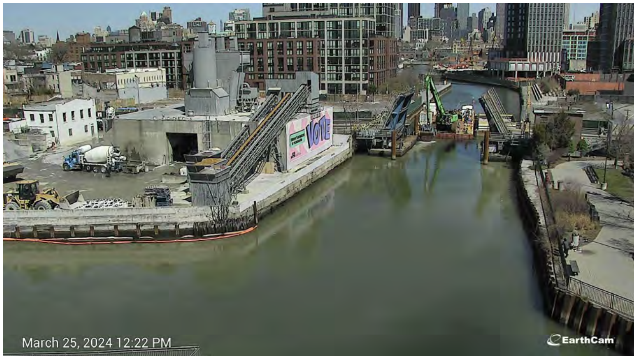
Figure 7. Visual indication of elevated turbidity as a result of gravel placement in and around Third Street Bridge at 12:15 PM on Monday, March 25, 2024.
