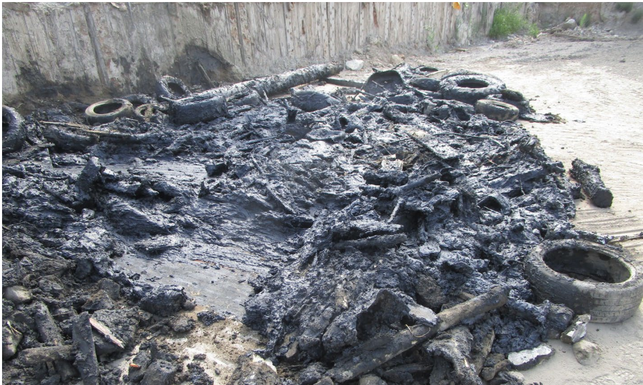
Photograph 1. An excavator was utilized to spread material out for inspection. Note high frequency of automotive tires and canal timbers (Chronicle Heritage, July 29, 2024).
