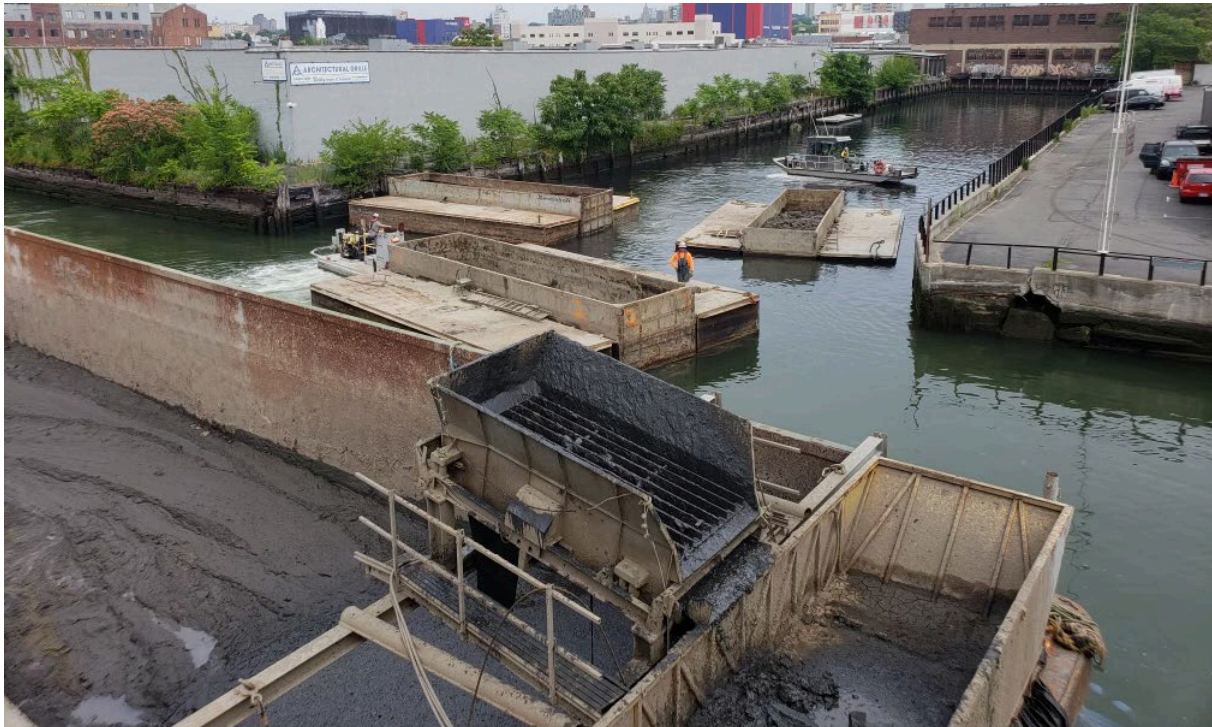
Photograph 2. PCB contaminated dredged soils are placed into shaker for removal of objects larger than 4-inches for Level 2 inspection by Chronicle Heritage (Cashman, August 9, 2024).
