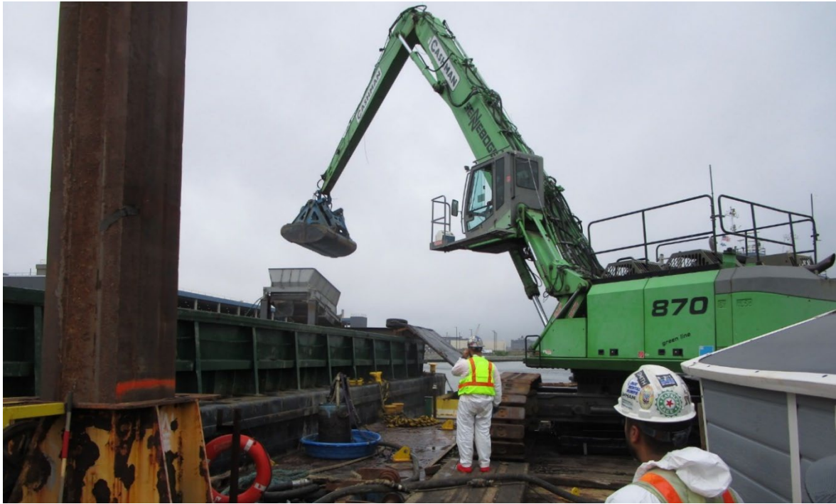
Photograph 1. PCB contaminated dredged soil being screened at Gowanus Canal Staging Area on August 9, 2024 (Chronicle Heritage, August 9, 2024).
