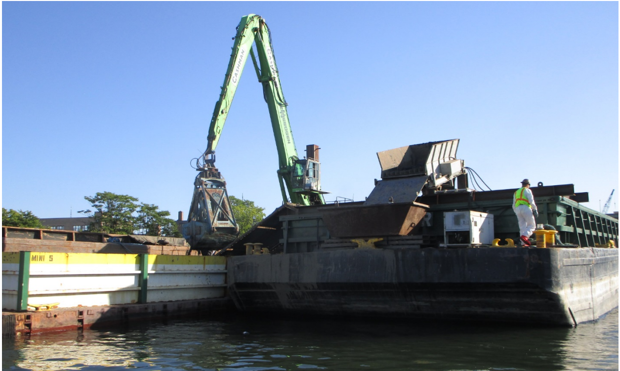
Photograph 1. PCB-contaminated dredged sediment being screened at Gowanus Canal Staging Area on August 12, 2024, facing southwest (Chronicle Heritage, August 9, 2024).
