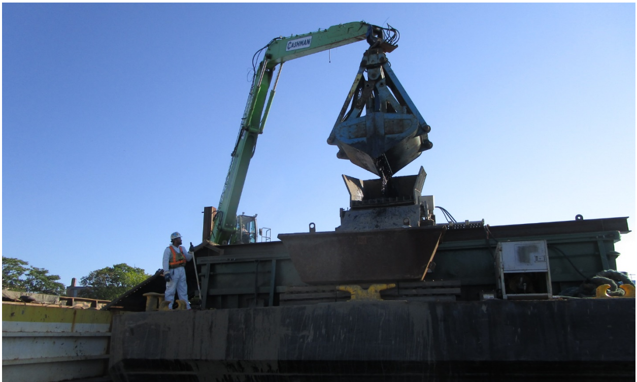
Photograph 2. PCB-contaminated dredged sediment being placed into a shaker for removal of objects larger than 4x8-inches for Level 2 inspection by Chronicle Heritage. Facing Southwest (Chronicle Heritage, August 12, 2024).
