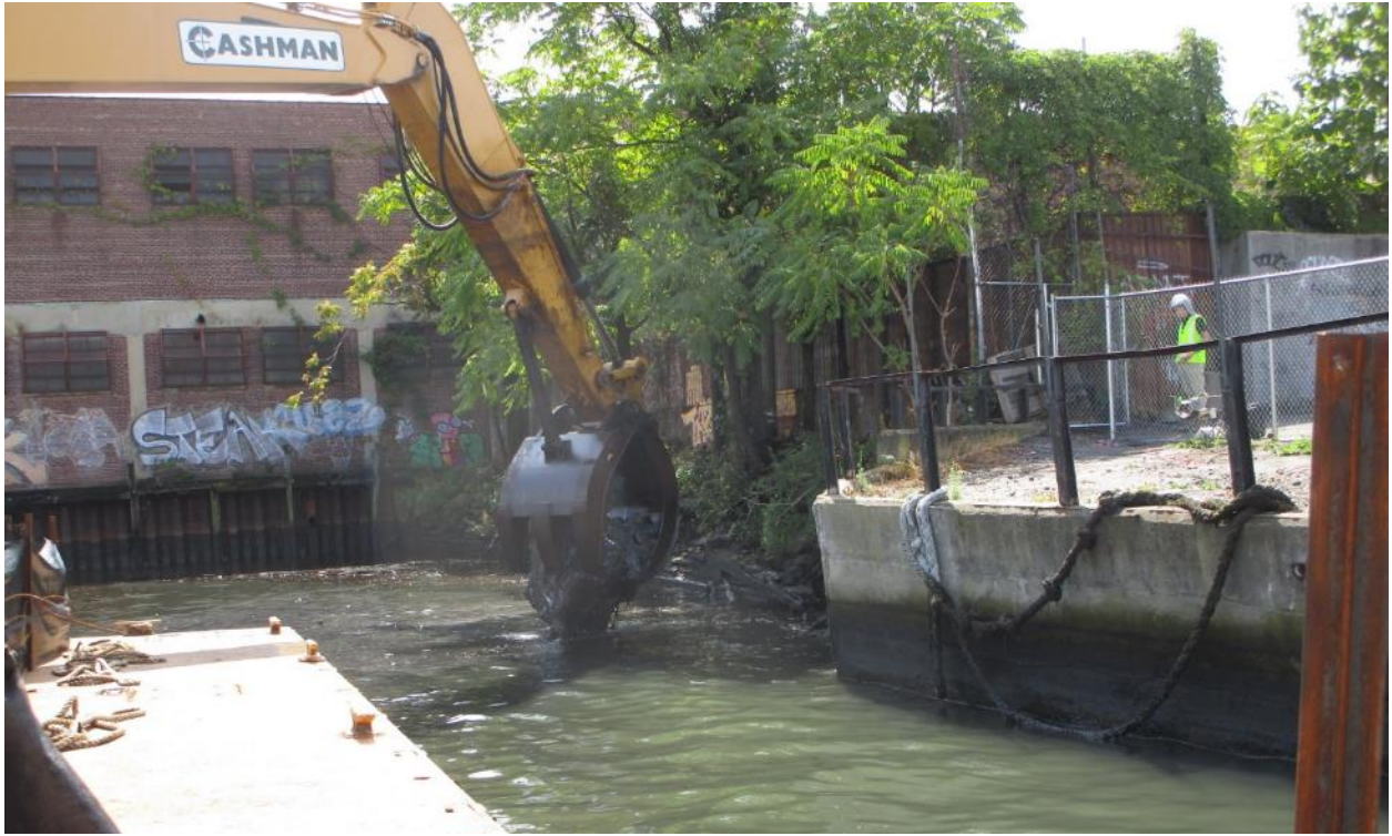
Photograph 2. Dredging periphery of Target 42b - removal of large concrete object, facing southeast (Chronicle Heritage, August 19, 2024).
