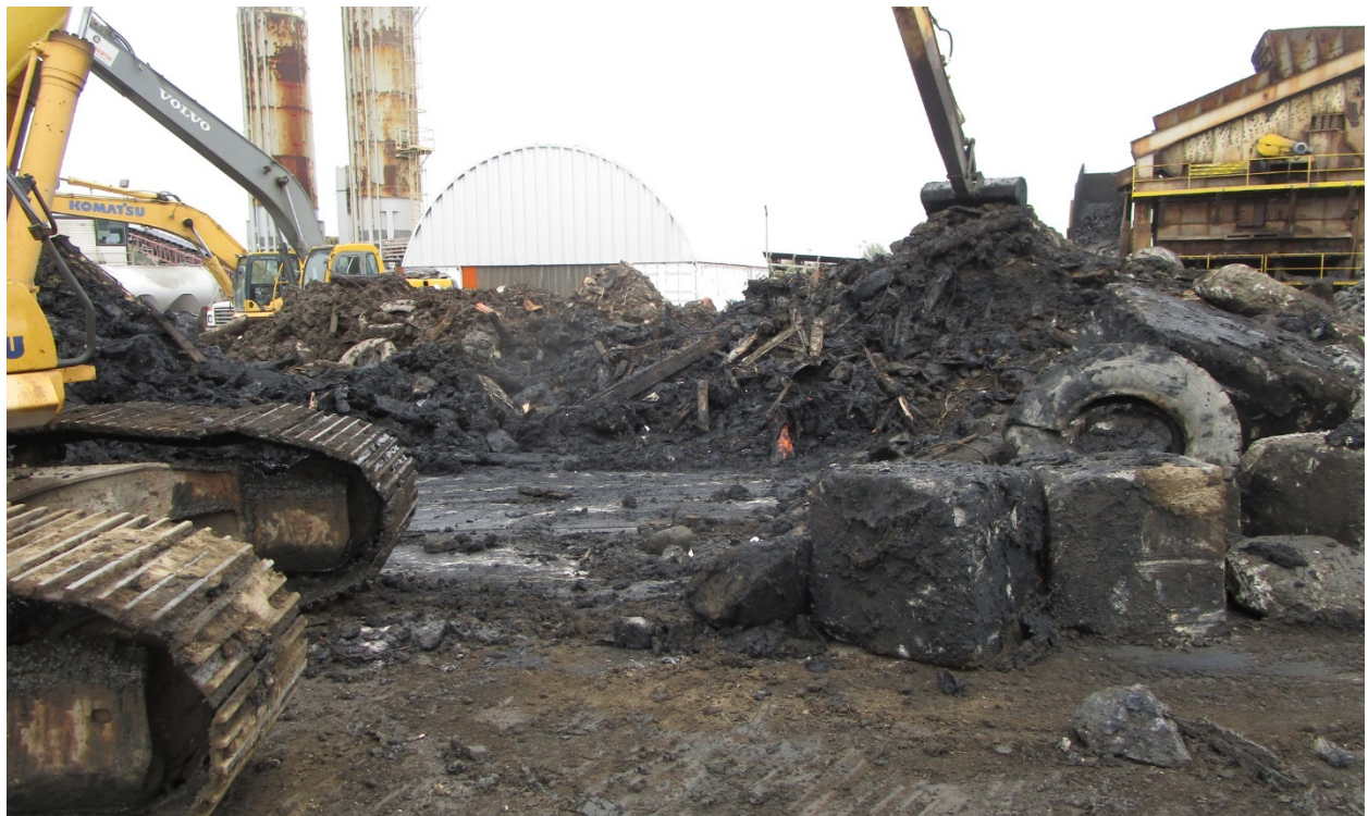
Photograph 2. An excavator was utilized to spread material out for inspection. Note high frequency of canal timbers, concrete blocks, rocks and tires (Chronicle Heritage, September 26, 2024).
