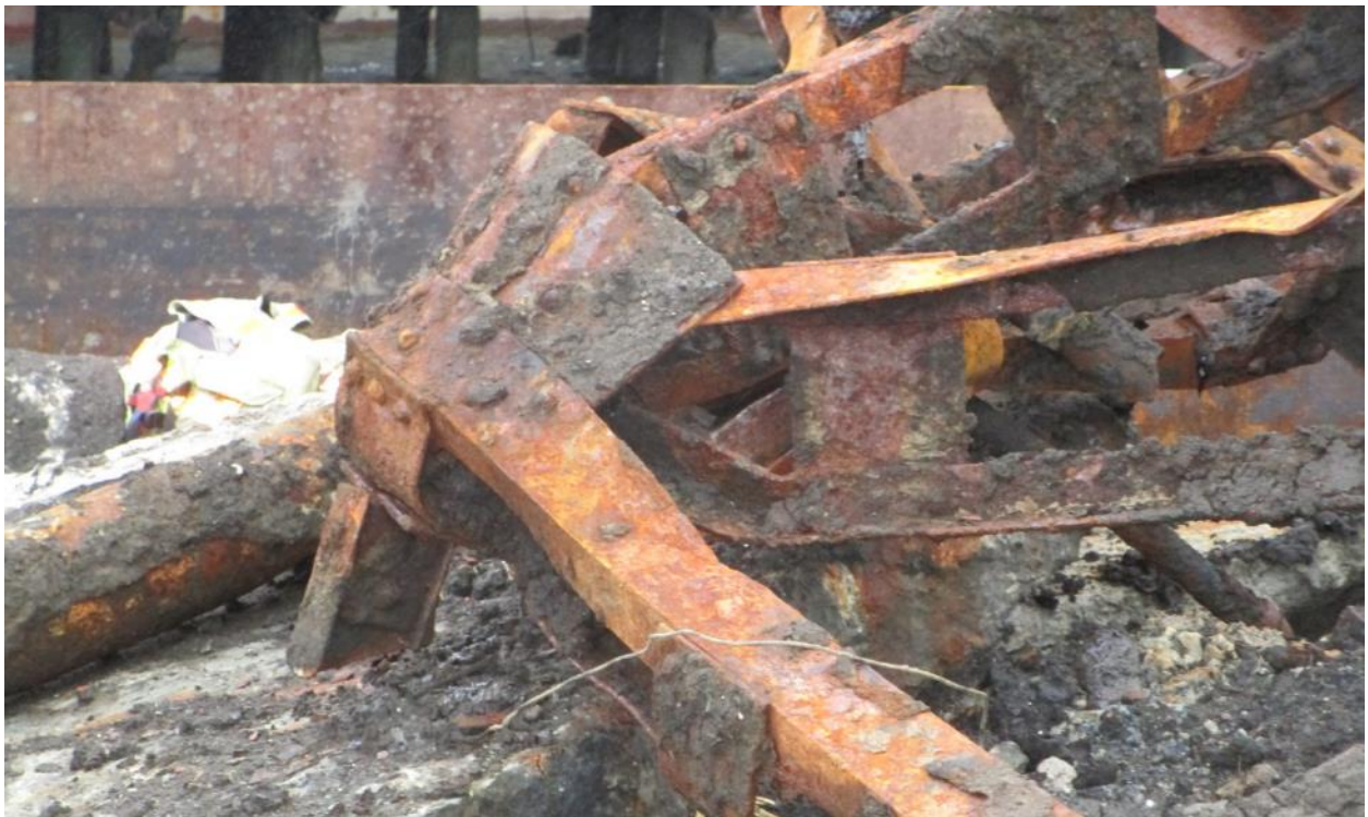
Photograph 3. Steel truss: Detail of angle iron and rivet construction (Chronicle Heritage, August 7, 2024).
