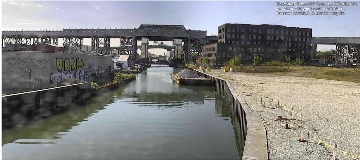
Figure 9– October 9, 2024. General Conditions in Canal looking towards 9 th Street Bridge at midday.
