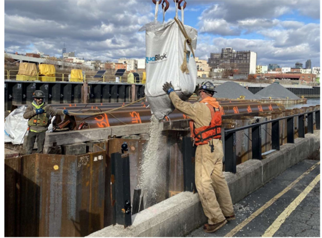
Contractors placing sealant around newly constructed bulkhead
