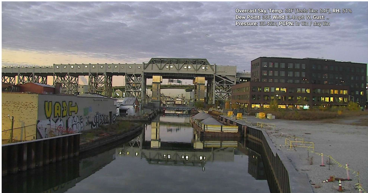
Figure 8 – October 28, 2024. General Conditions in Canal looking towards 9 th Street Bridge prior to work activities. Slight sheen noted.
