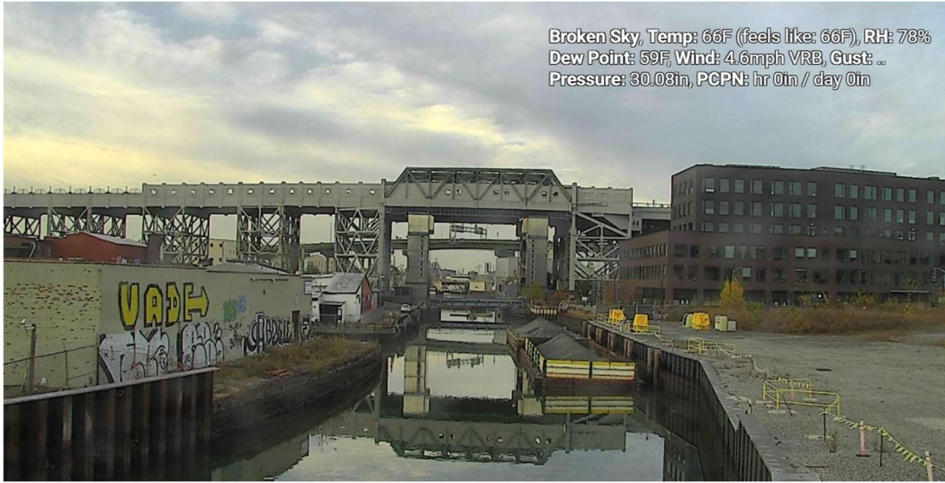
Figure 10 – November 8, 2024. General Conditions in Canal looking towards 9 th Street Bridge prior to work activities. Slight sheen noted.
