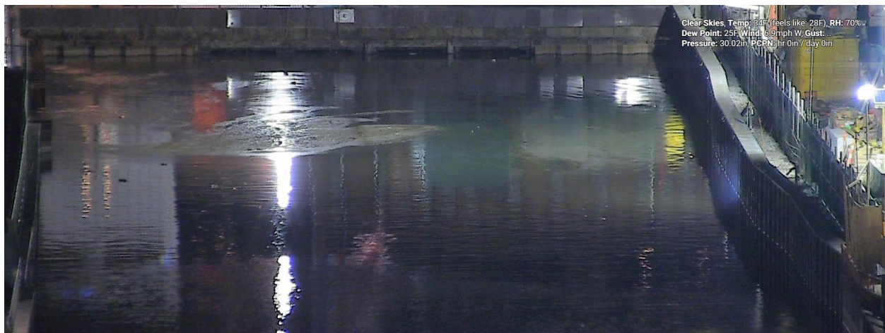
Figure 11 -January 13, 2025. After rain overnight, CSO discharges were noted at the headwall.
