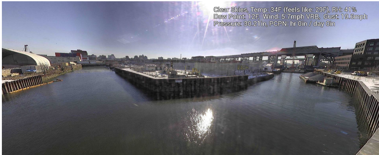
Figure 8 – January 24, 2025. General Conditions in Canal north of 9 th Street Bridge during in-waterway construction activities.
