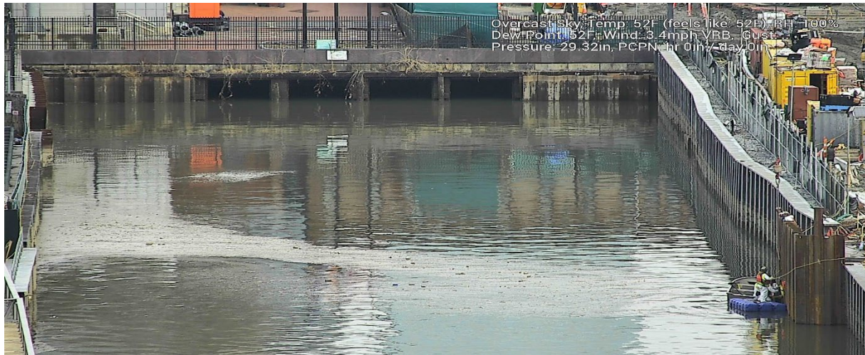
Figure 11- March 6, 2025. Conditions at the headwall of Canal showing increased floatables at 8:52 AM.
