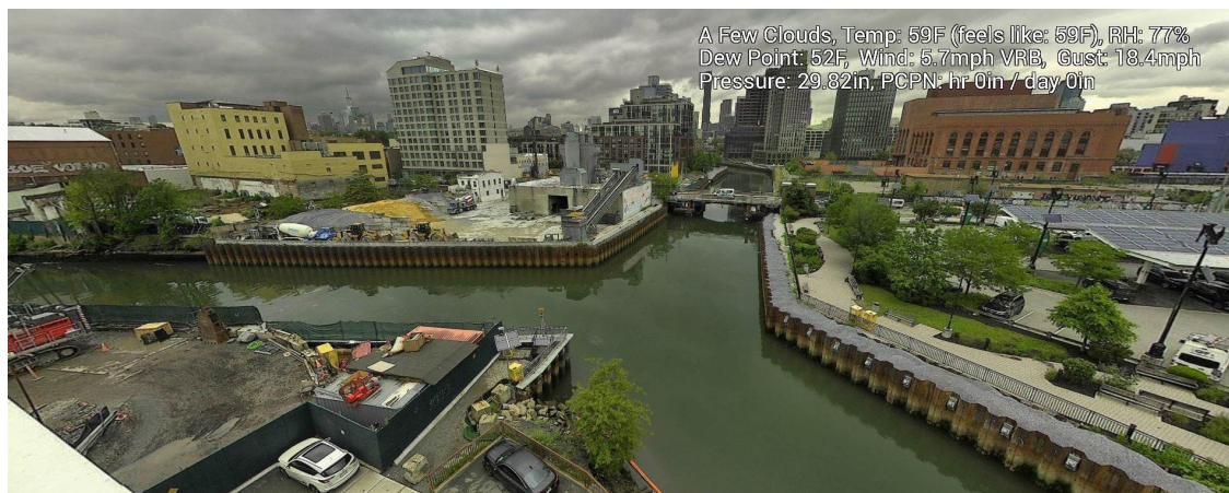
Figure 10 – May 23, 2025. General Conditions in Canal south of 3 rd Street Bridge near TB4 during in-waterway construction activities.
