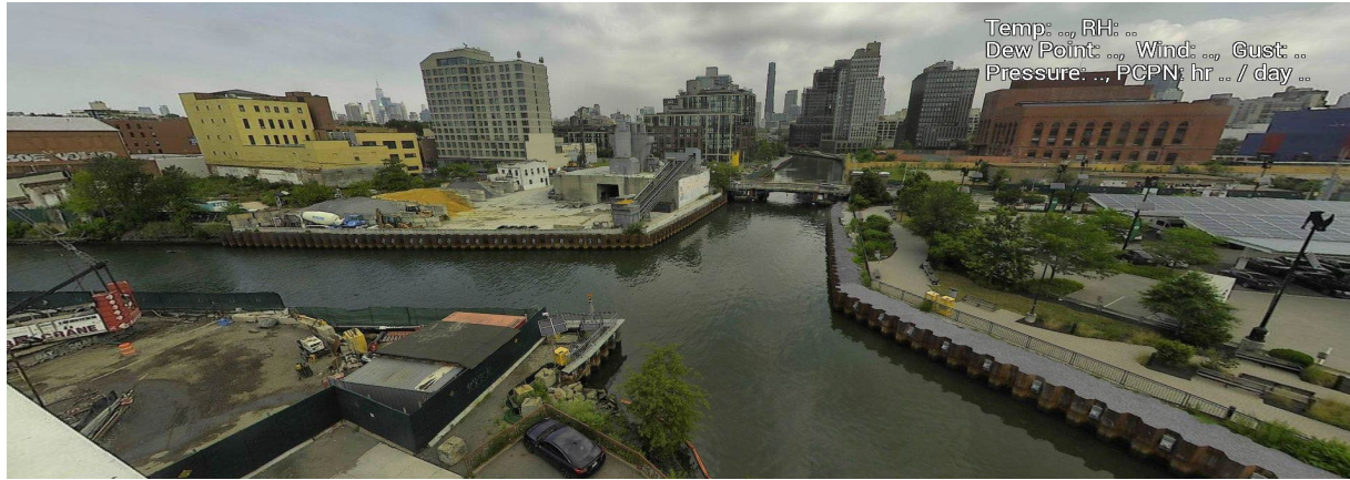
Figure 10 – July 11, 2025. General Conditions in Canal south of 3 rd Street Bridge near TB4 during in-waterway construction activities.
