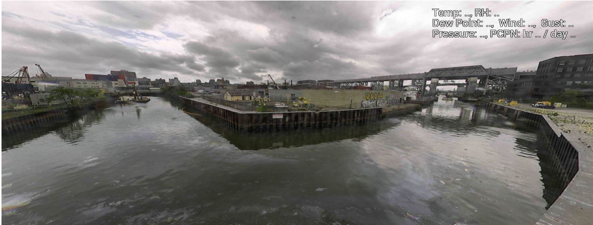
Figure 8 – July 7, 2025. General Conditions in Canal north of 9 th Street Bridge near TB6 during in-waterway construction activities.
