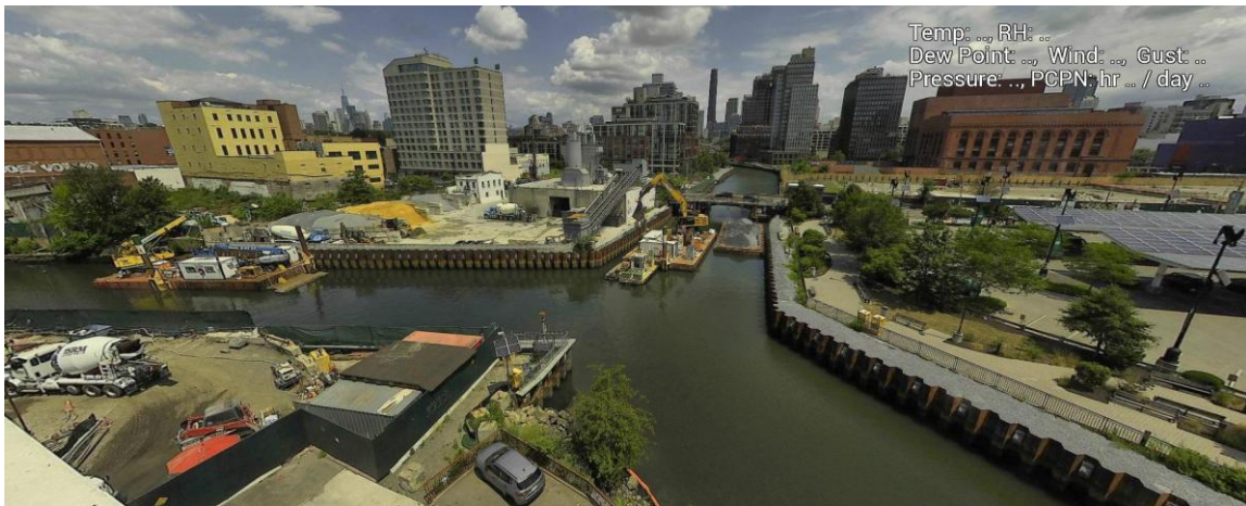
Figure 9 – July 23, 2025. General Conditions in Canal south of 3 rd Street Bridge near TB4 during in-waterway construction activities.
