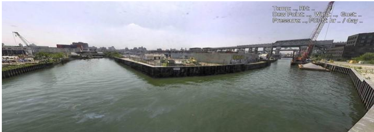
Figure 10 – July 25, 2025. General Conditions in Canal north of 9 th Street Bridge near TB6 during in-waterway construction activities.
