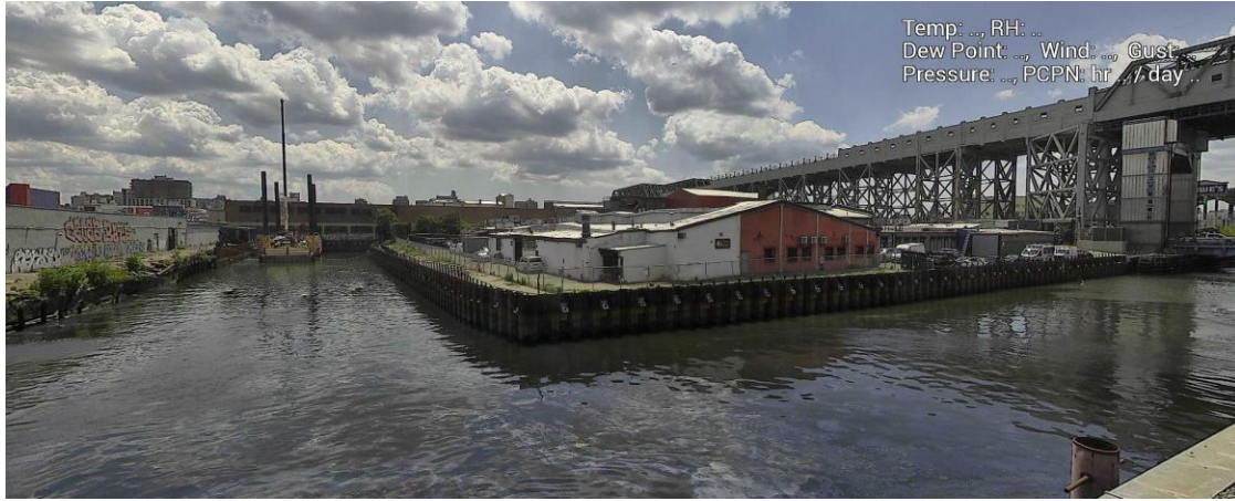
Figure 8 – July 21, 2025. General Conditions in Canal north of 9 th Street Bridge near TB7 during in-waterway construction activities.
